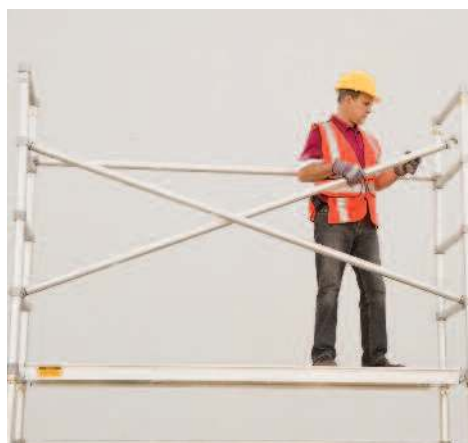
2. Snap horizontal and then diagonal braces in place.
