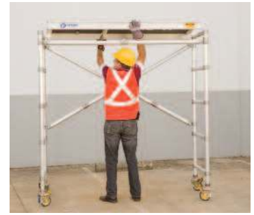
4. Install platform at desired height.
