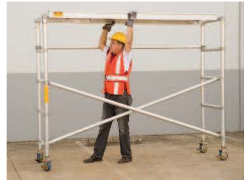
3. Install platform at desired height.
